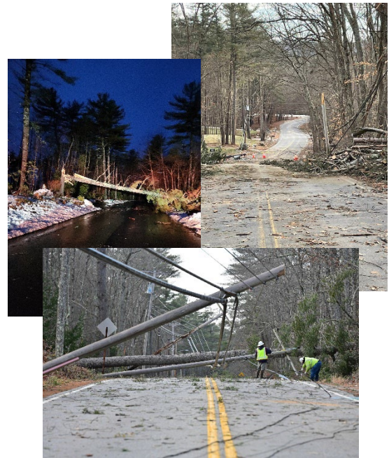
Figure 3 – Damage caused by Winter Storm Elliot
